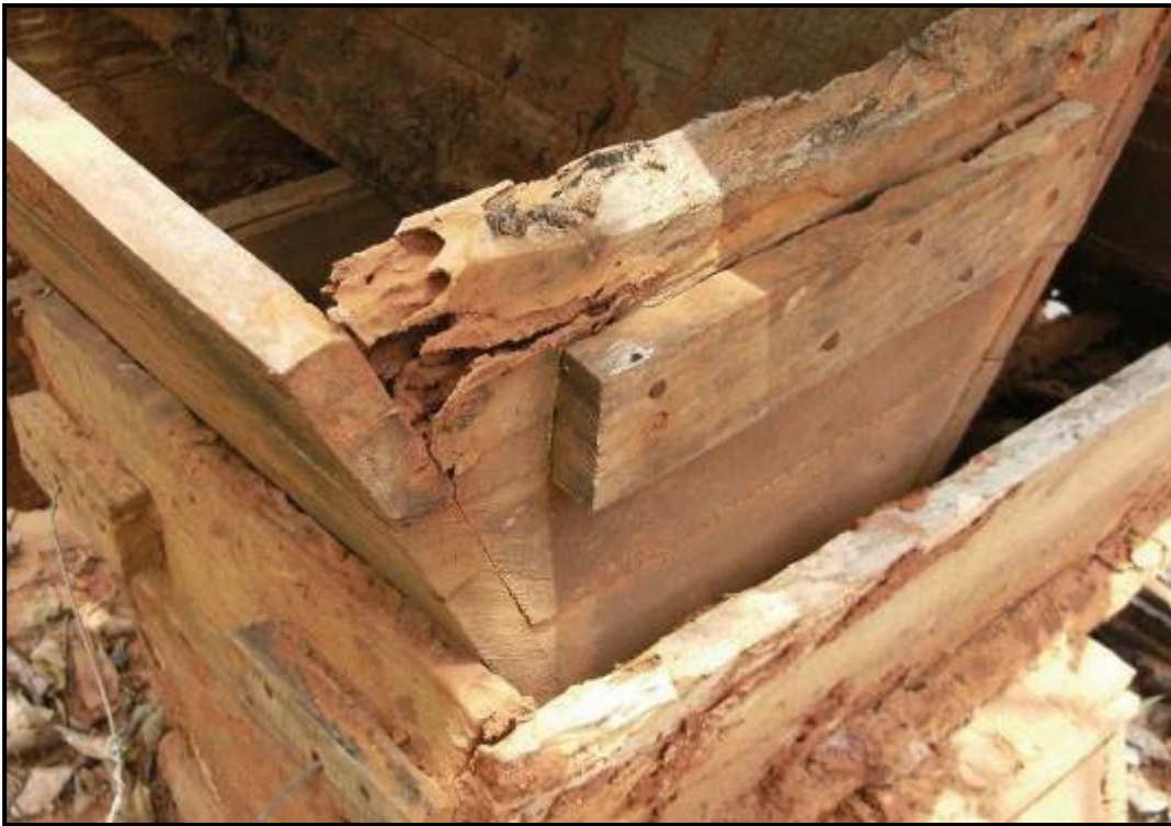
Termite damage.
