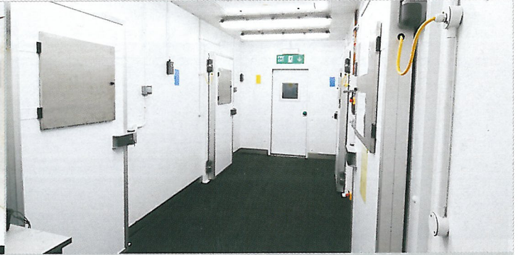
Figure 4. The cold corridor of the QEU, maintained at a temperature of -15\text{ }^{\circ}\text{C}
