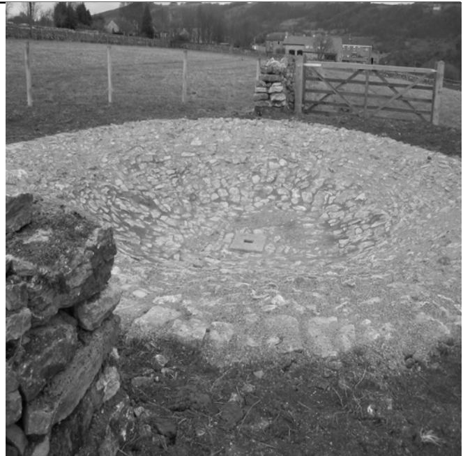
Restored clay and stone sett dew pond
